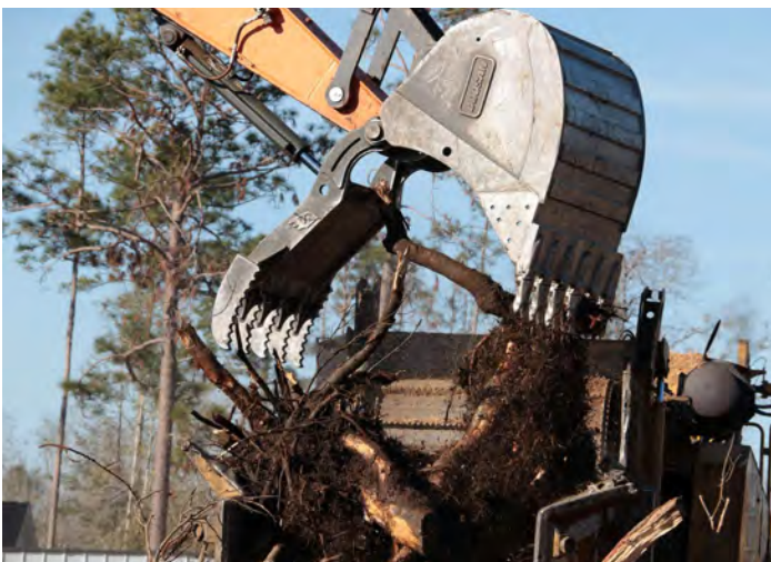
Clean up after Hurricane Michael a 2018 Category 5 storm that brought wind gusts in the 60-75+ mph range to Georgia, downing countless trees and power lines.
